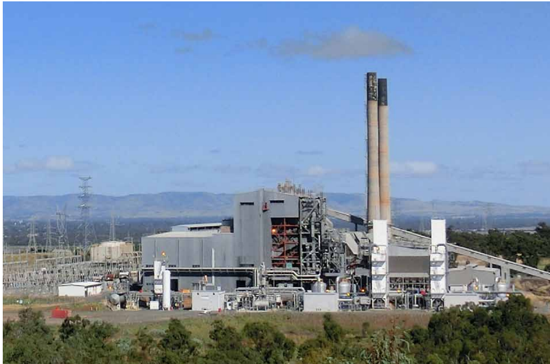
The site of the Callide Oxyfuel Project – Callide A Power Station in Central Queensland, Australia.
